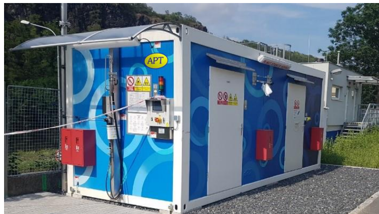
Small hydrogen fueling station in ÚJV Řež
